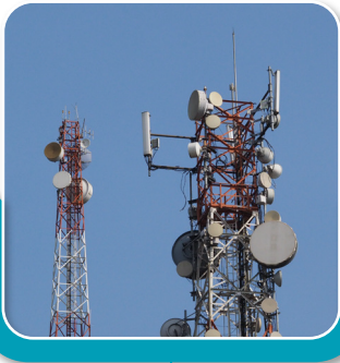
ANTENNA BASE STATION
